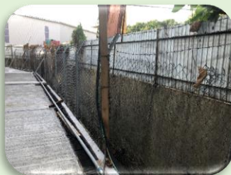
After Removal Works 雜草清除工作後
