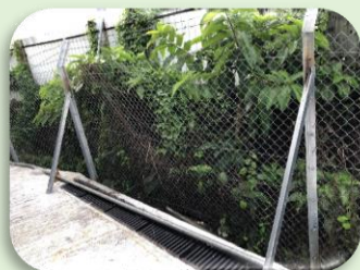
Before Removal Works 雜草清除工作前
